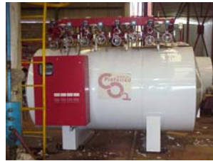
Low Pressure CO2 Bulk Tank Installation.jpg
